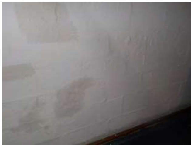
EFFLORESCENCE
